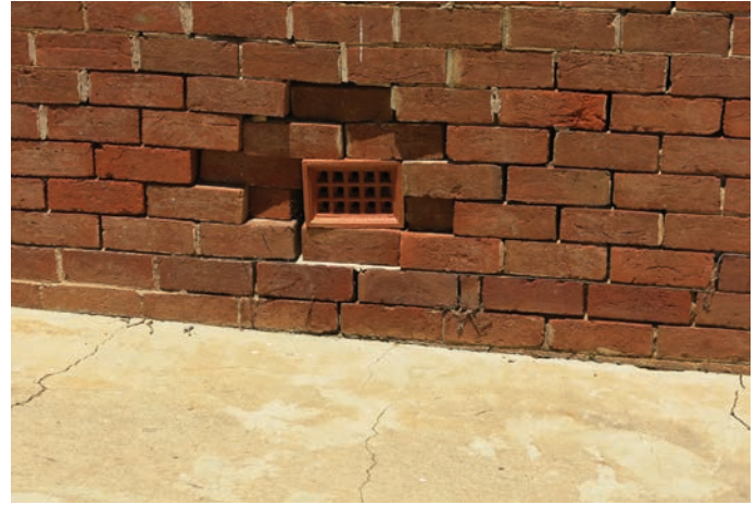
Loss of mortar and loose air vents make it easy for insects to enter a building.
