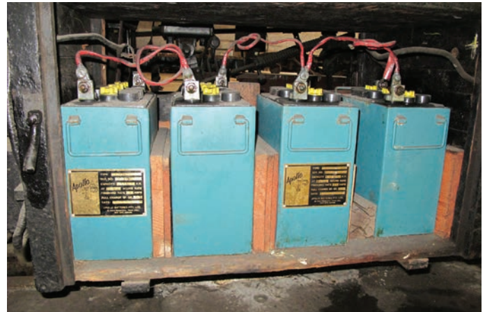
Remove batteries to stop acid leaks and corrosion.
